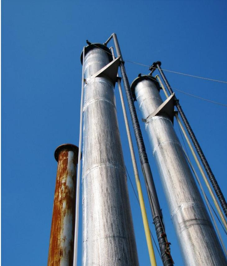
*Purification towers clean the gas to at or above pipeline standards.*
