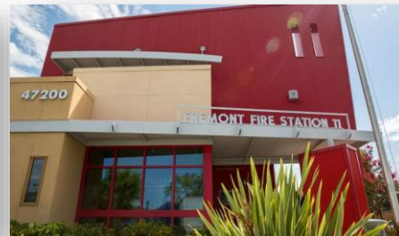
City of Fremont Fire Station
