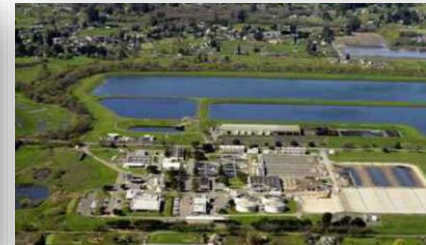
Laguna Waste Water Treatment Plant
